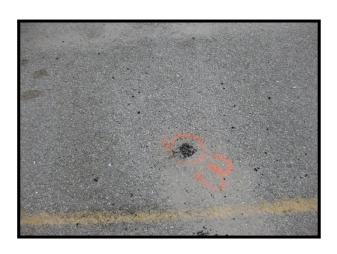
Photo: Each temporary monitor well was purged until the purge water was free and clear of sediment. Samples were collected and the location was restored with asphalt patch.
