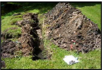
Photo: Test trenches were excavated along the northern and western areas of the Pond identified as the former landfill. The test trenches were advanced to at least the top of the water table and inspected for evidence of buried solid waste.
