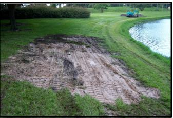
Photo: Once the test trenches were complete and observations noted, four representative soil samples were collected and then the areas were restored.
