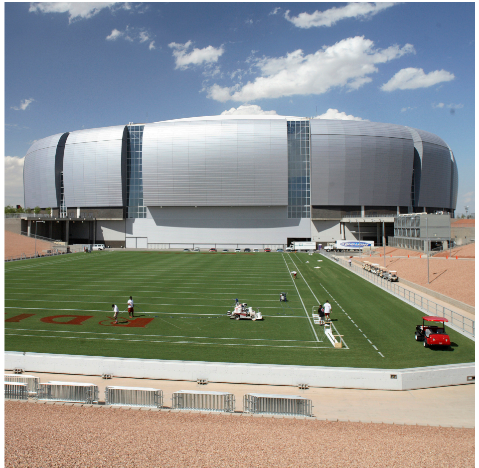
credit: University of Phoenix Stadium
